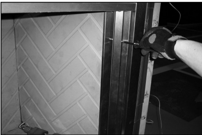
Figure 12.3 Loosen Refractory Retaining Strip
